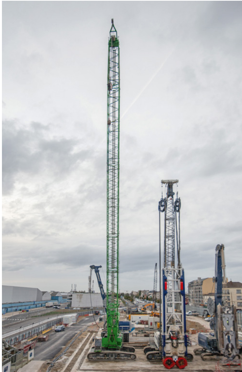
The first contract for Line 17 was awarded at the beginning of the year. This 439.4 million euro contract covers the works for package 1, between Le Bourget and Gonesse. Construction of the underground walls of Le Bourget Aéroport station began in fall of 2019.
