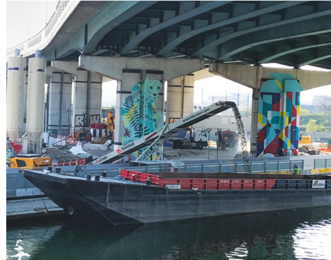
River platforms were built to load barges with spoil directly from the worksites. The first transfer took place in spring on the Puits du Canal worksite in Aubervilliers. Alternative forms of transportation for spoil removal on the Grand Paris Express became a reality in 2019.
