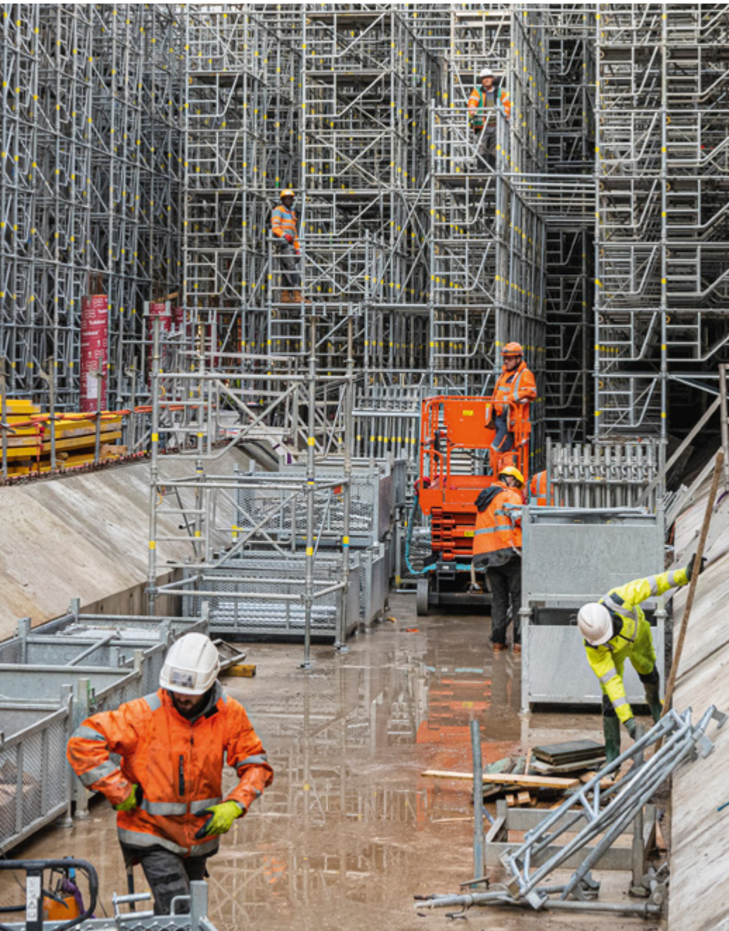
The Grand Paris Express worksites marked their one millionth hour of work integration in summer 2019 thanks to the ramp-up of construction, mainly on Lines 15 South and 16. Over 1,600 people have signed work integration contracts since works started.
