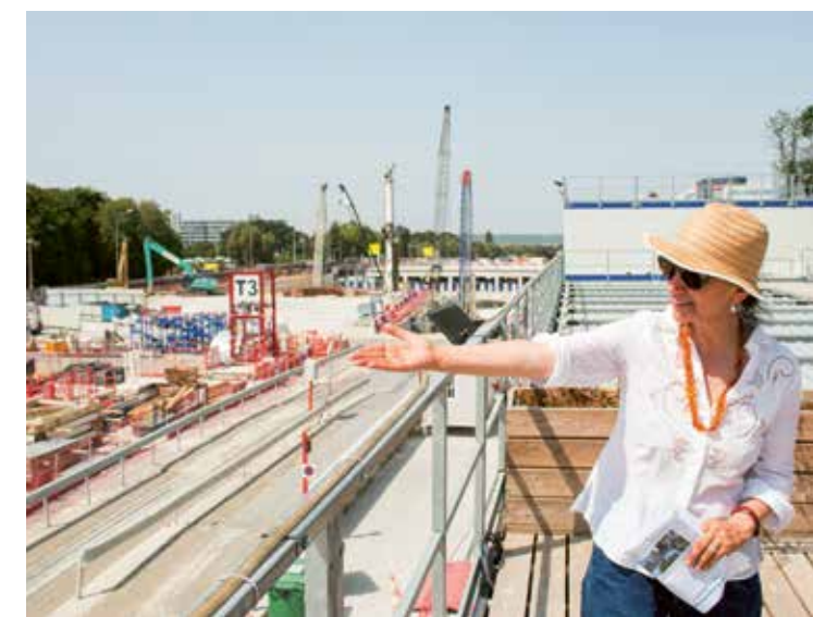
Tour guide Carmen Atias tells visitors about the Noisy - Champs station worksite at the field office.
